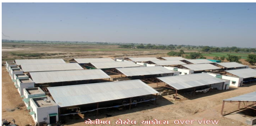
A hostel for Cattle in Akodara, Gujarat
